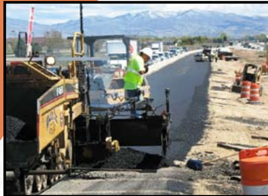
I-84 Eagle Westbound Off-ramp
