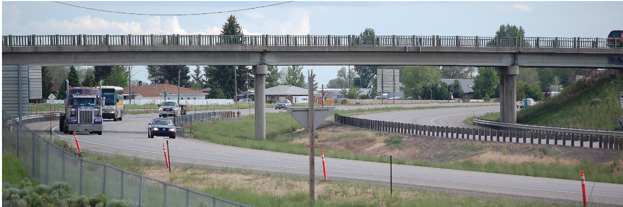
Pancheri Overpass on I-15 south of Idaho Falls.
