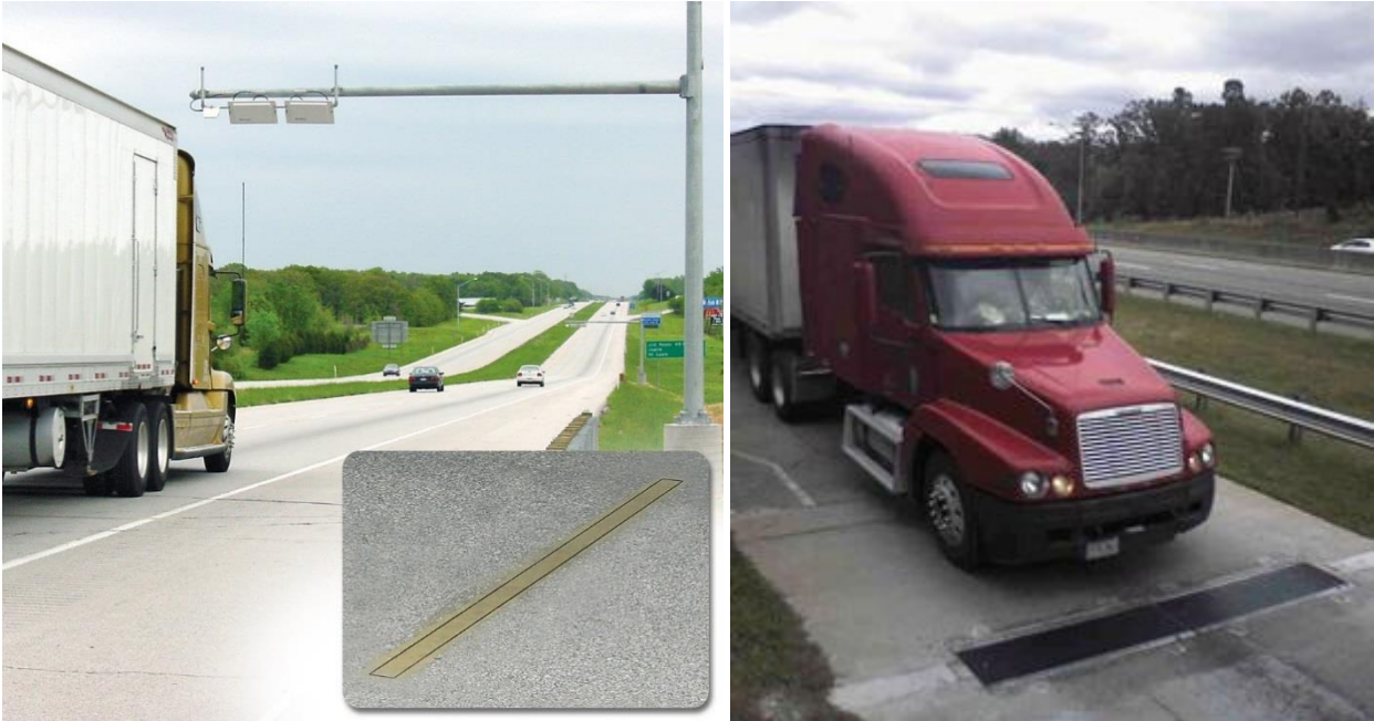
Figure 24. Photo of Quartz Sensor (Left) and Bending Plate (Right)
