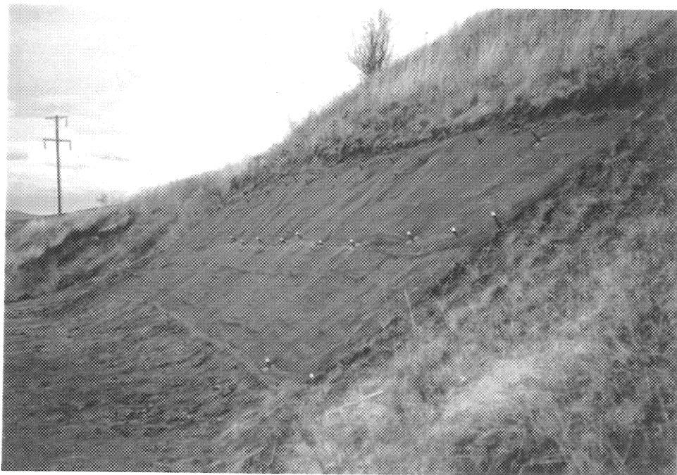
Figure 2. Geogrid-backed, synthetic erosion control blanket after hydroseeding treatment and post-tensioning of soil pins; test site on US 95 south of Moscow.
