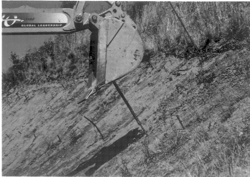
Figure 1. Installation of soil pins (No. 6, threaded steel rebar) using a backhoe bucket and driving sleeve; test site on US 95 south of Moscow.
