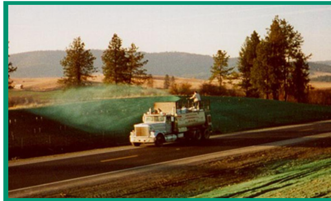
Hydroseeding project demonstration on Highway 9 between Deary and Princeton: a slurry of native plant seed and wood fiber mulch.
