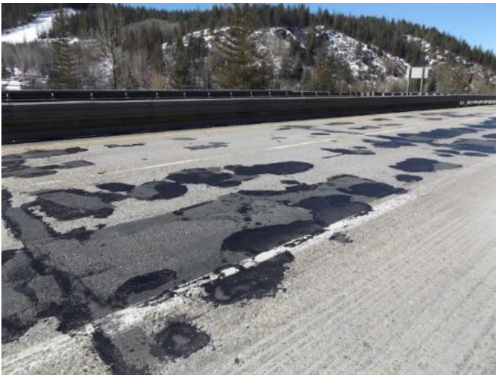
Photo 5-4: Example of Poor Condition Bridge Deck
