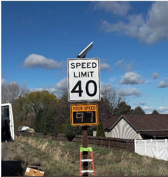
Adjusted speed zone limits and added speed feedback signs/speed limit ahead signs with beacons for driver awareness.
