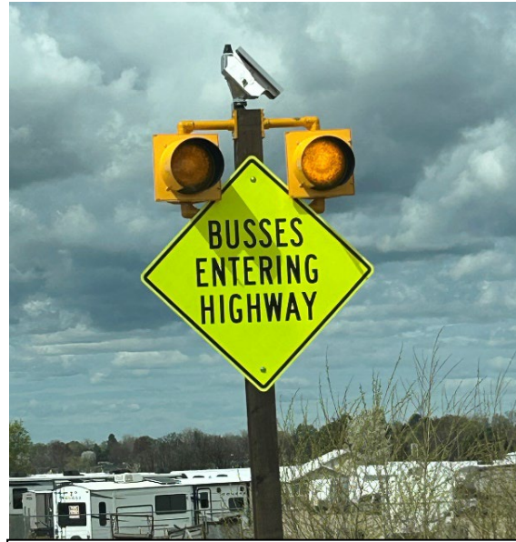
Enhanced bus safety signage with flashing beacons near Emmett's PRRTA technical high school on SH-16.
