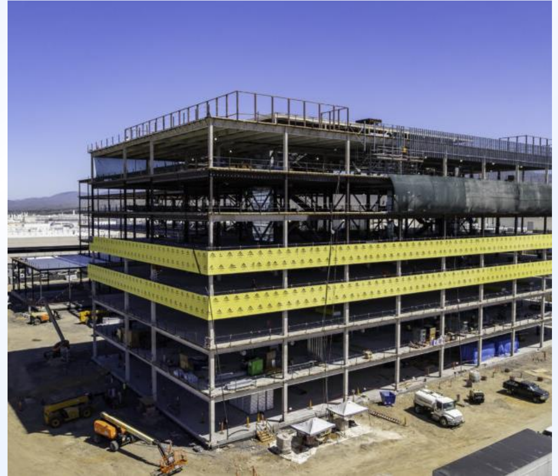
Micron's chip facility under construction in east Boise. Source: Idaho Business Review
