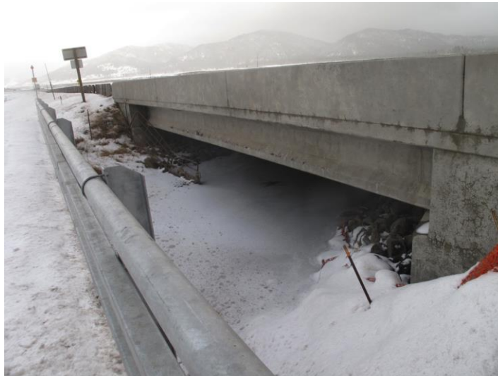
Figure 56. US-20 MP 398.67 Henrys Lake Outlet Bridge
