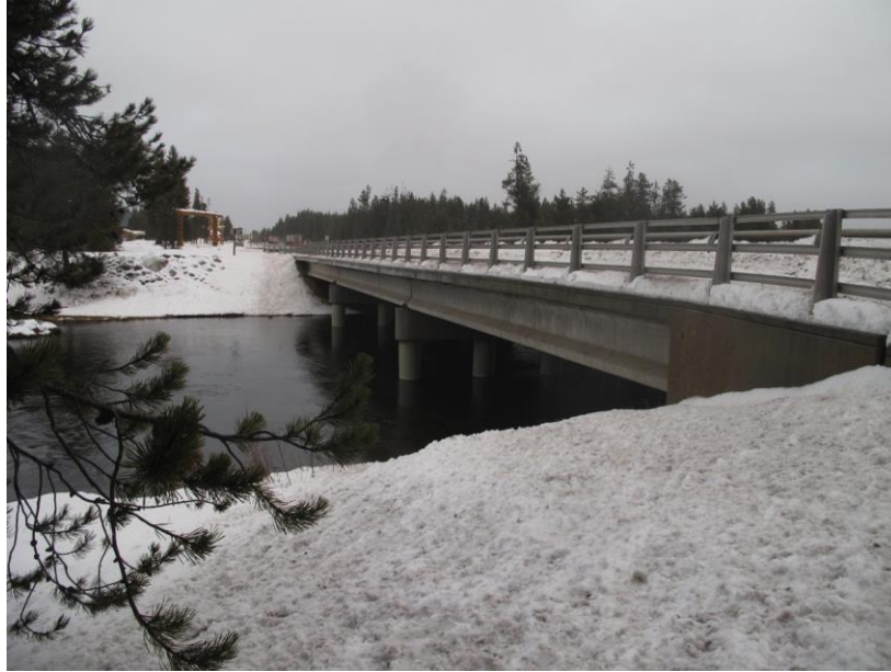
Figure 54. US-20 MP 387.04 Ponds Lodge/Henry's Fork Bridge
