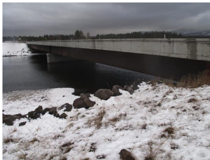
Figure 53. Osborne Bridge, US-20 MP 379
