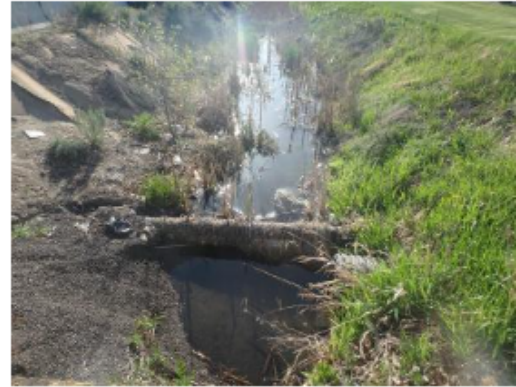
Drainage swale(s). Click the image to enlarge
