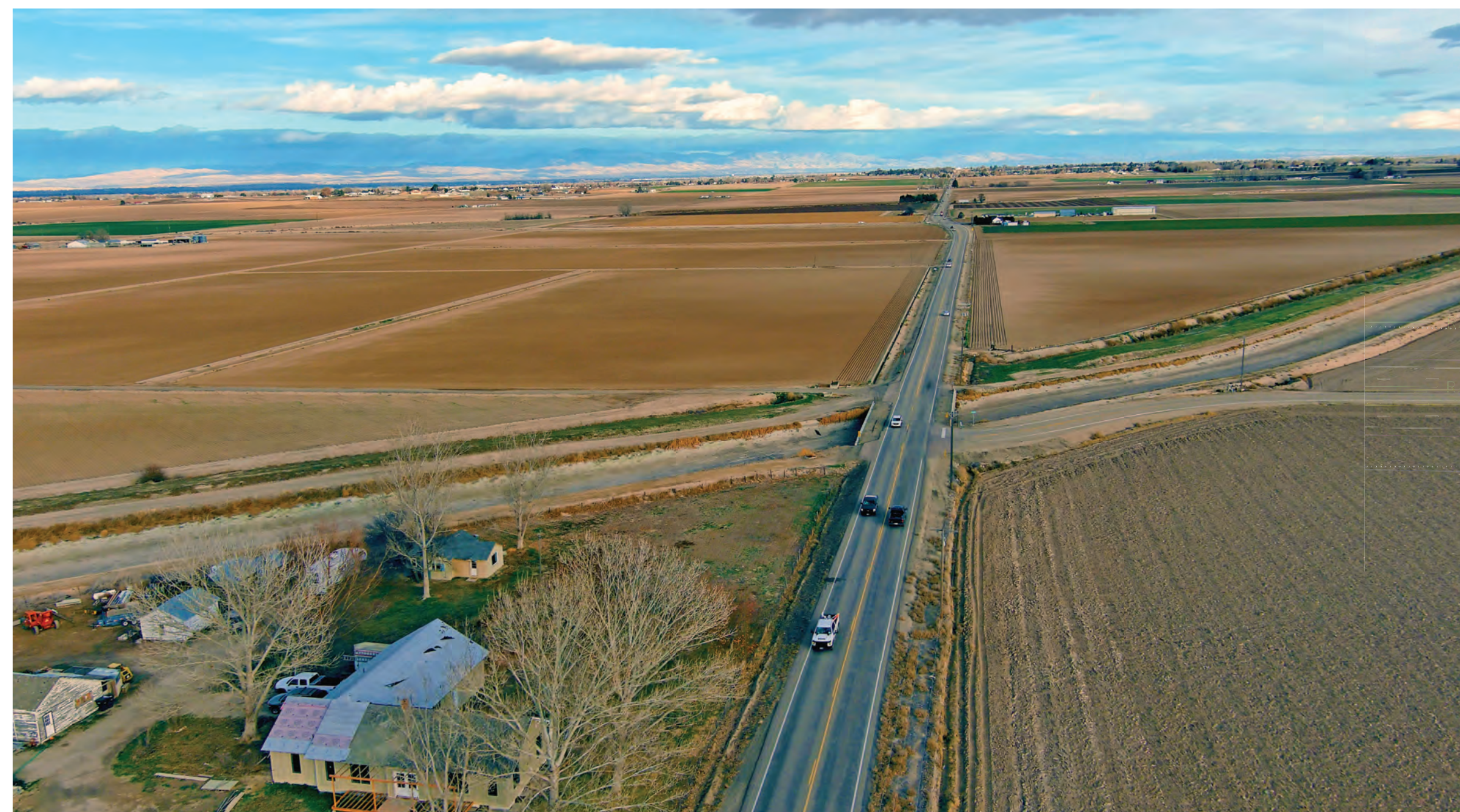
Intersection of SH-55 and Pecan Lane
