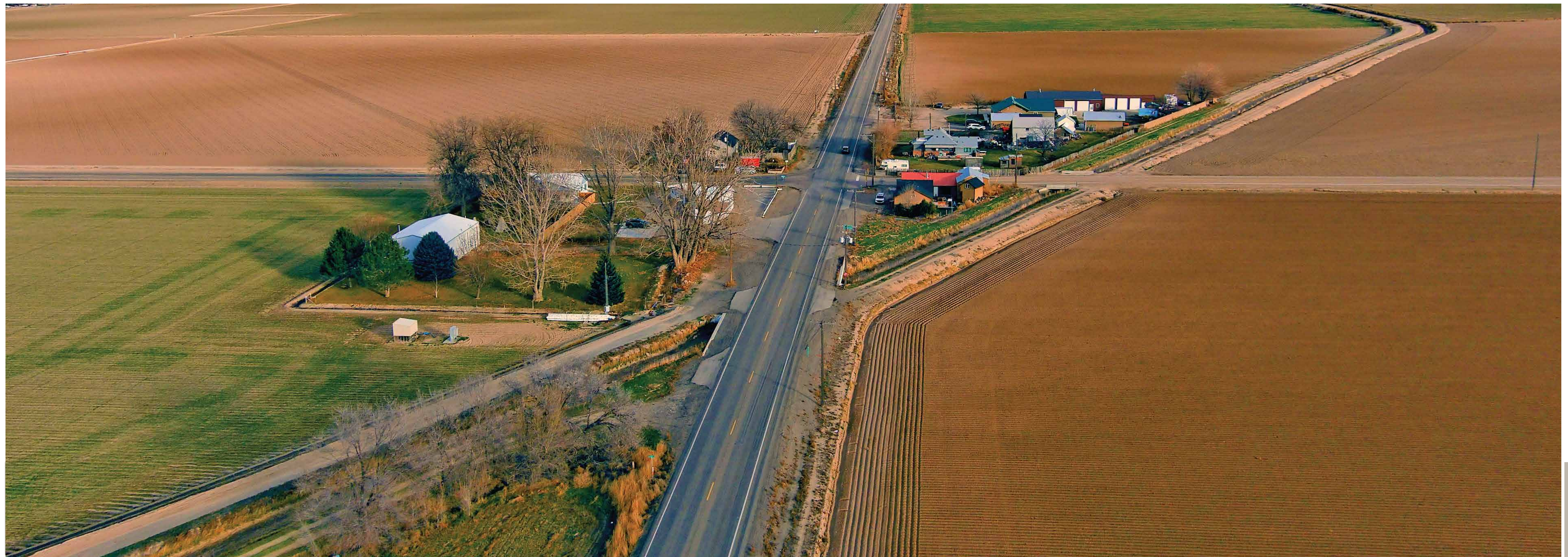
Canal crossing at the intersection of SH-55 and Pride Lane
